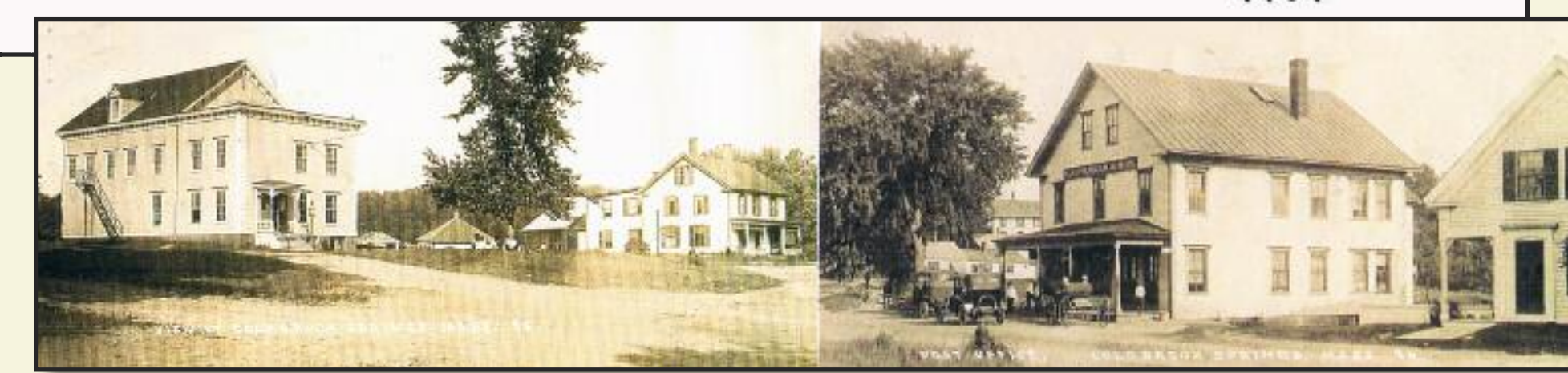
Main Street looking east
